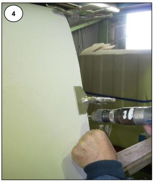
cut-out position by placing tube off-cut against panel and marking rail. See Photos 7 & 8.
