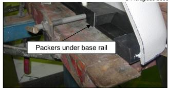
21 Carefully bend the outer rail around the rear corner, clamp and rivet in place. See Photo 24. Note: There may be an enlarged gap between the rail upstand and canopy bottom around the corner; this can be reduced by driving it inwards using a wooden block struck with a hammer or directly using a soft faced mallet.
